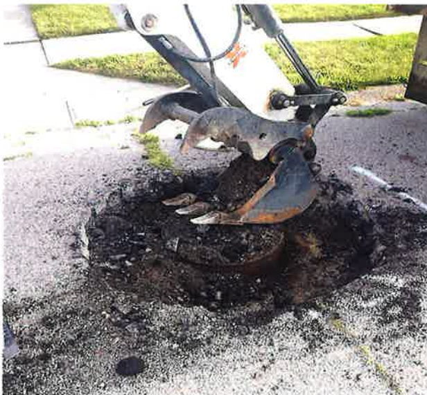
The Service crew repaired a sanitary manhole on Ankara Avenue, the concrete under the metal casting had failed.
