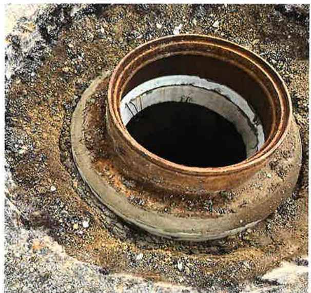
The Service crew repaired a sanitary manhole on Ankara Avenue, the concrete under the metal casting had failed.
