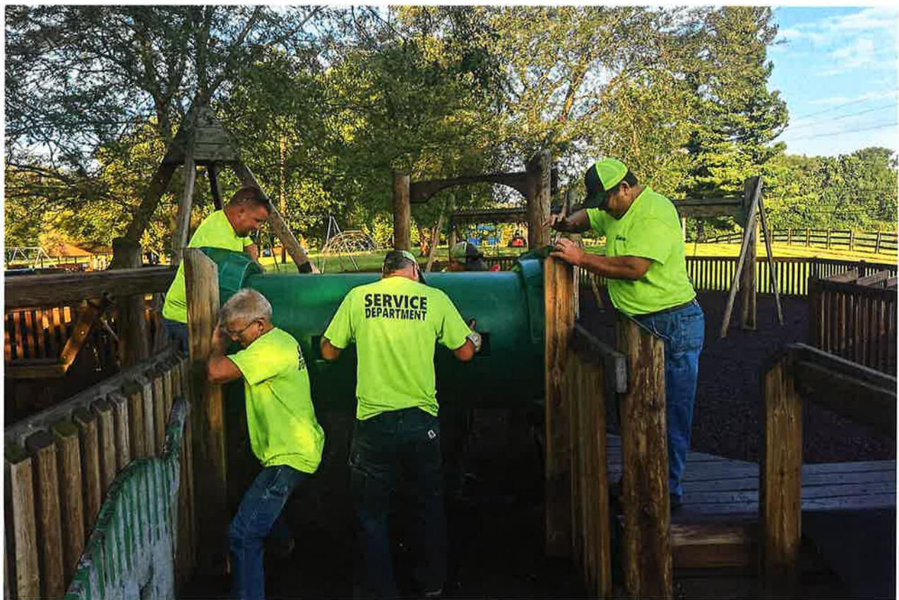
In September 2021, the Service Department replaced a damaged crawl tube in the Castle Playground. The old tube had cracked, leaving dangerous sharp edges. The new tube was purchased by the Brookville Chamber of Commerce.
