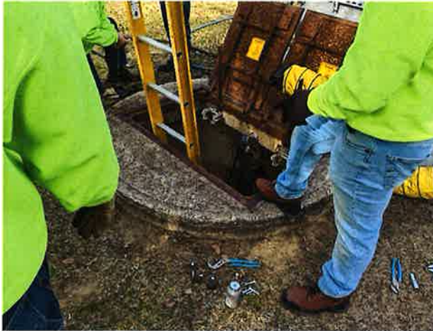
The Service Department performs rehab work on the Urban Lane lift station, replacing the guide rails for the pumps.
