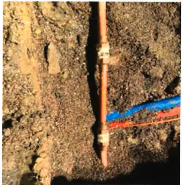
The above picture shows a water service that was hit by a directional boring machine. Service crews removed the damaged section of copper and repaired the line.
