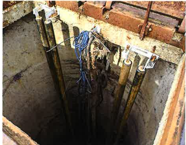
The Service Department performs rehab work on the Urban Lane lift station, replacing the guide rails for the pumps.
