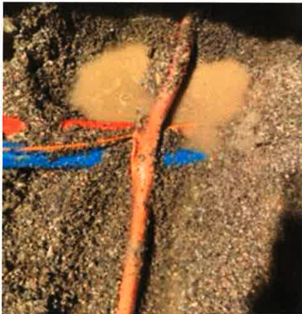
The above picture shows a water service that was hit by a directional boring machine. Service crews removed the damaged section of copper and repaired the line.
