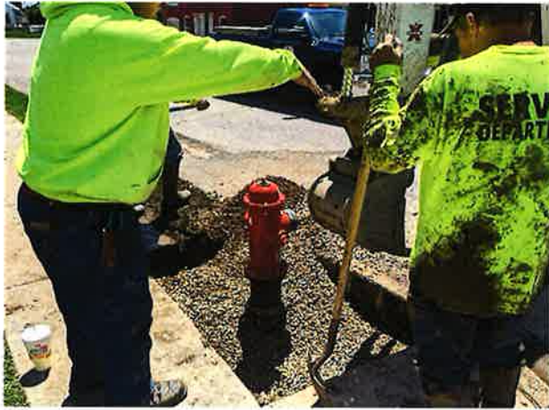
Fire Hydrant replacement on Jefferson St.
