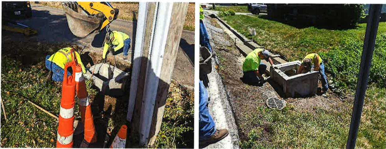
The picture above shows a new catch basin set in place and the curb restored to match the existing. After the concrete cures, the Service Department will remove the forms, reset the cast iron lid, and patch the asphalt.
