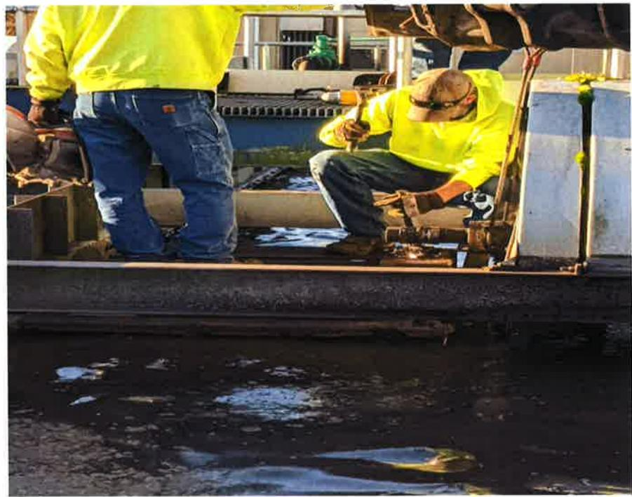
The Wastewater Treatment Plant uses a Vertical Loop Reactor (VLR) to help airate the wastewater, supporting the growth of aerobic bacteria. The Service Department had to replace a broken shaft on one of the VLR's in 2020. A crane was used to help reset the shaft after the turning vanes were transferred to the replacement shaft.
