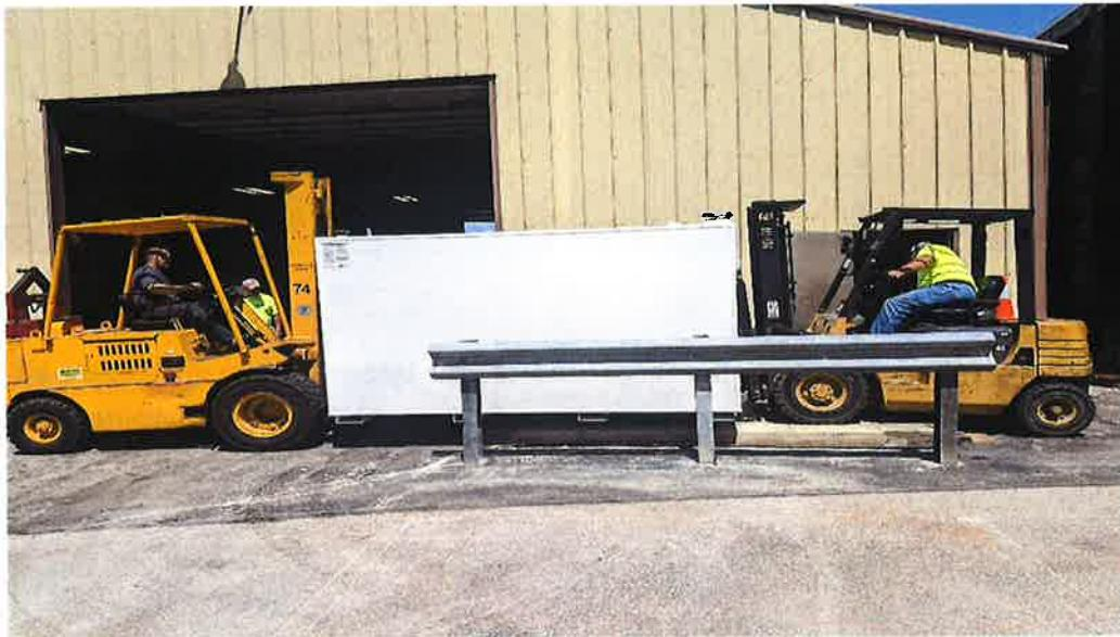
The Service Department received a grant for a new used oil tank in 2020. This tank has double-wall protection. The tank can hold 1,400 gallons of used oil for the waste oil furnace that heats the Service Garage. Personnel are installing the new used oil tank above.
