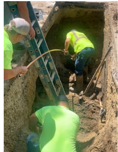
E. Westbrook Water line switchover
